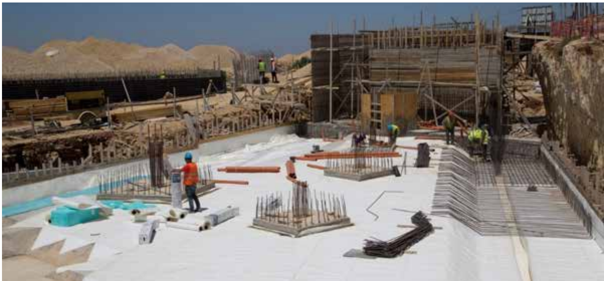
Figure 12: Installing insulation material
