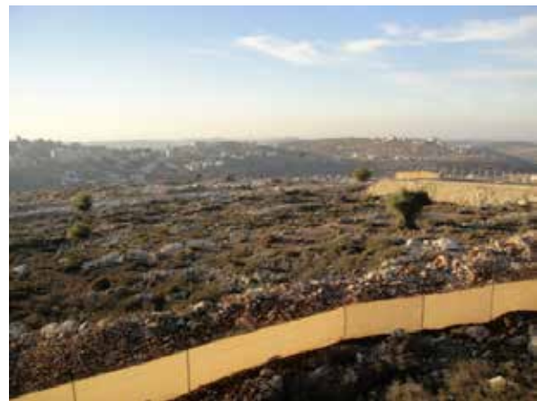
Figure 3: Silt fence
