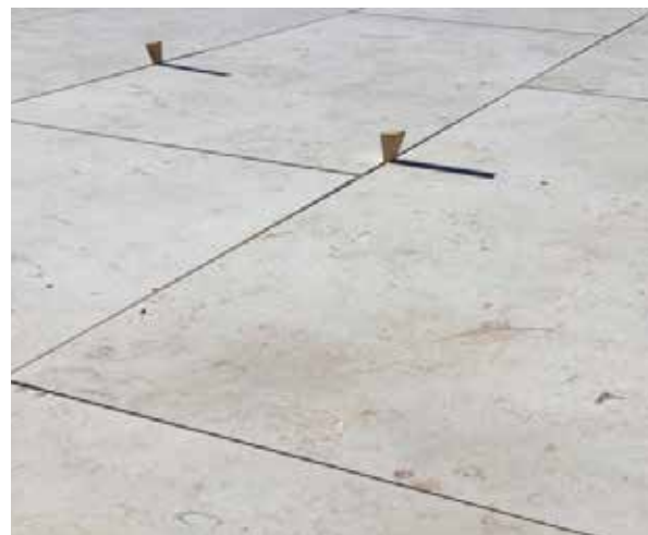
Figure 10: Untreated white stone used for the roof area
