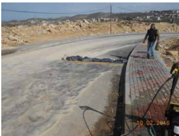
Figure 2: Sandbag barrier at the site
