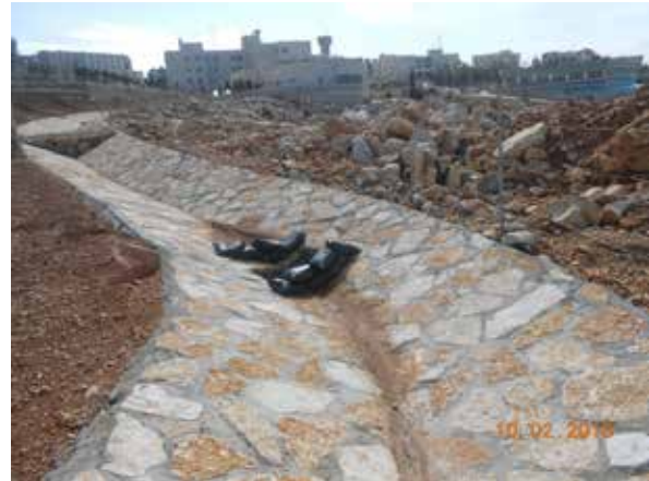
Figure 9: The swale - storm water management
