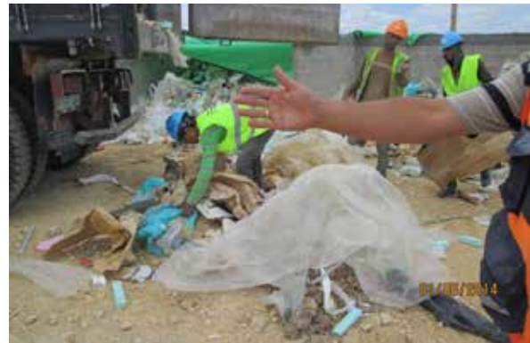
Figure 16: Construction waste management facility - LEED Laborers collecting the construction waste
