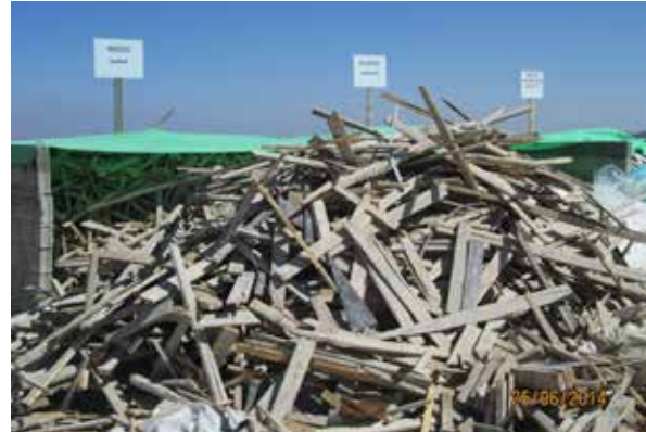
Figure 14: Construction waste management area - wood waste
