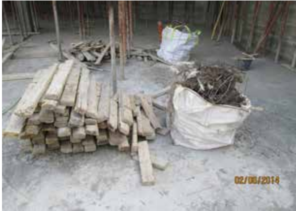
Figure 18: Steel and wood recyclable materials collection
