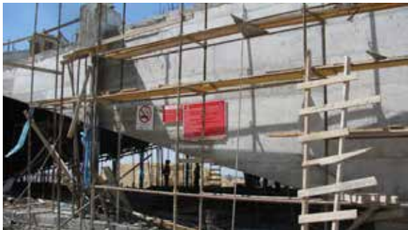
Figure 22: No Smoking signage
